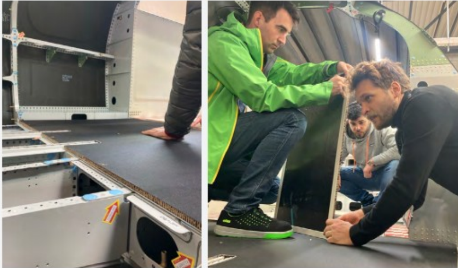
Trial fitting of floor panels built by German supplier, Diehl
